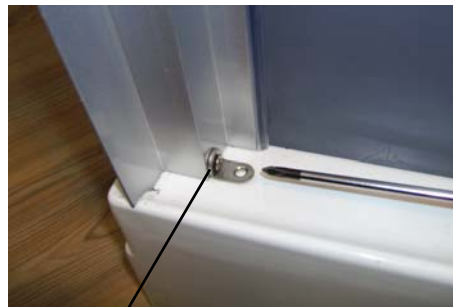
Použit šrouby 4,2x12 Svislé profily spojit s vaničkou use screws 4,2x12, link the vertical profiles with shower tray
