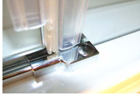
Zakrýt záslepkou cover with blind flange
