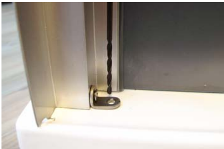
Vaničku vrtat vrtákem 3,2 mm drill the shower tray with 3,2mm drill
